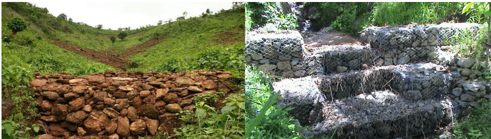
Gambar 6.14. Dam penahan susunan batu
